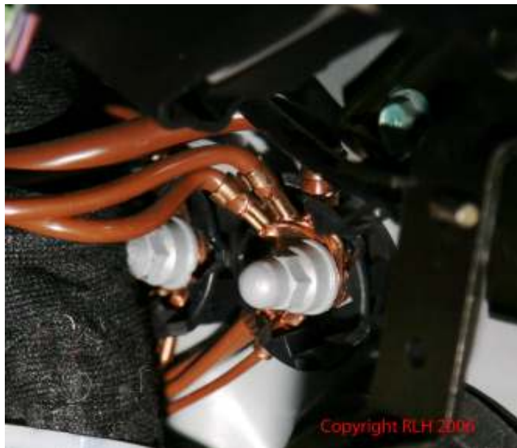
Photo 26 Typical Ground Stud
