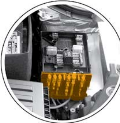
Electrical Box, In the Engine Compartment, Left Side
