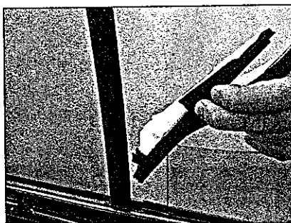
13.19b ... then slide upwards out of the guide rail
